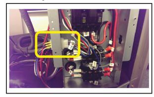
Fig. 15 – Connect J39 Plug Into P39 Connector Route the EH Harness to E-Box
