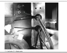
Fig. 12 – Routing Red and Black Wires
